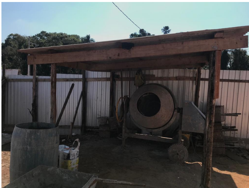
Figura 05 – Betoneira protegida contra as intempéries
